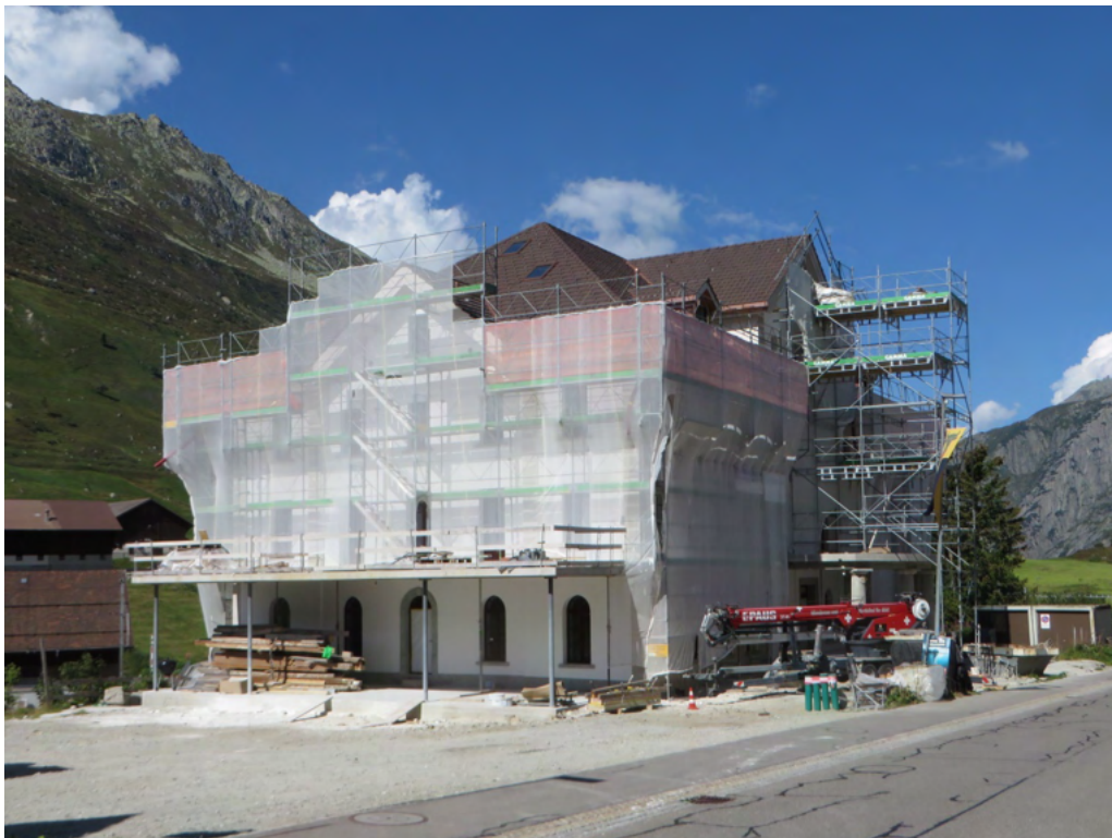
Renovation des Meyerhofs in Hospental am 5. September 2021.
